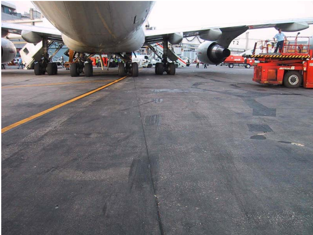
Ground marks the day of the incident (intermittent and strongly marked)
