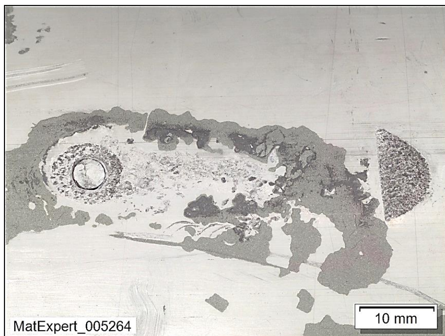
Figure 32: Area around joint 16/116 – pre-existing broken rivet and impact wear, erosion and cavitation on the spar tube.
