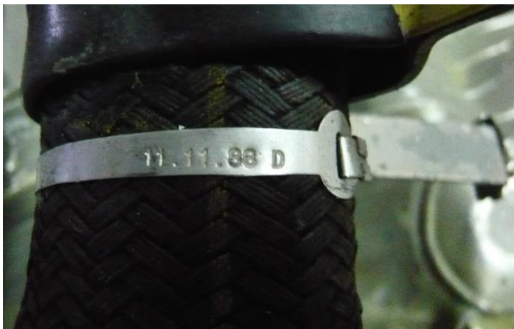
Figure 31: Hardened fuel line dated 11 November 1988.
