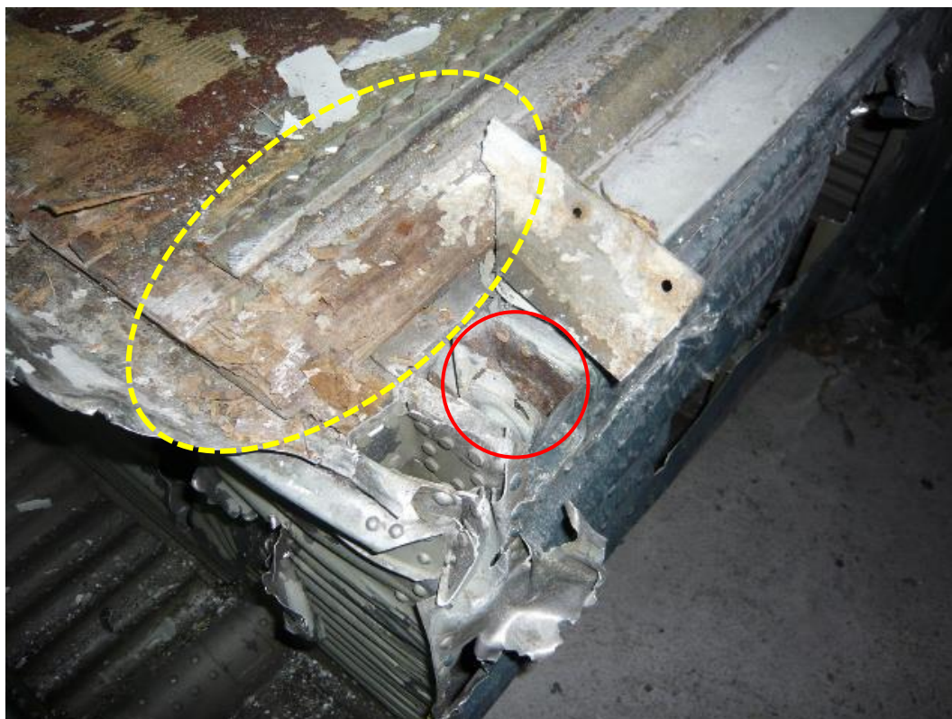
Figure 5: Close-up of figure 2 number (3) – rotten wooden floor (zone marked in yellow), severely corroded hinge of the cargo door (red circle) and severe corrosion on the fuselage structure (powdery, whitish patches of aluminium oxide).
