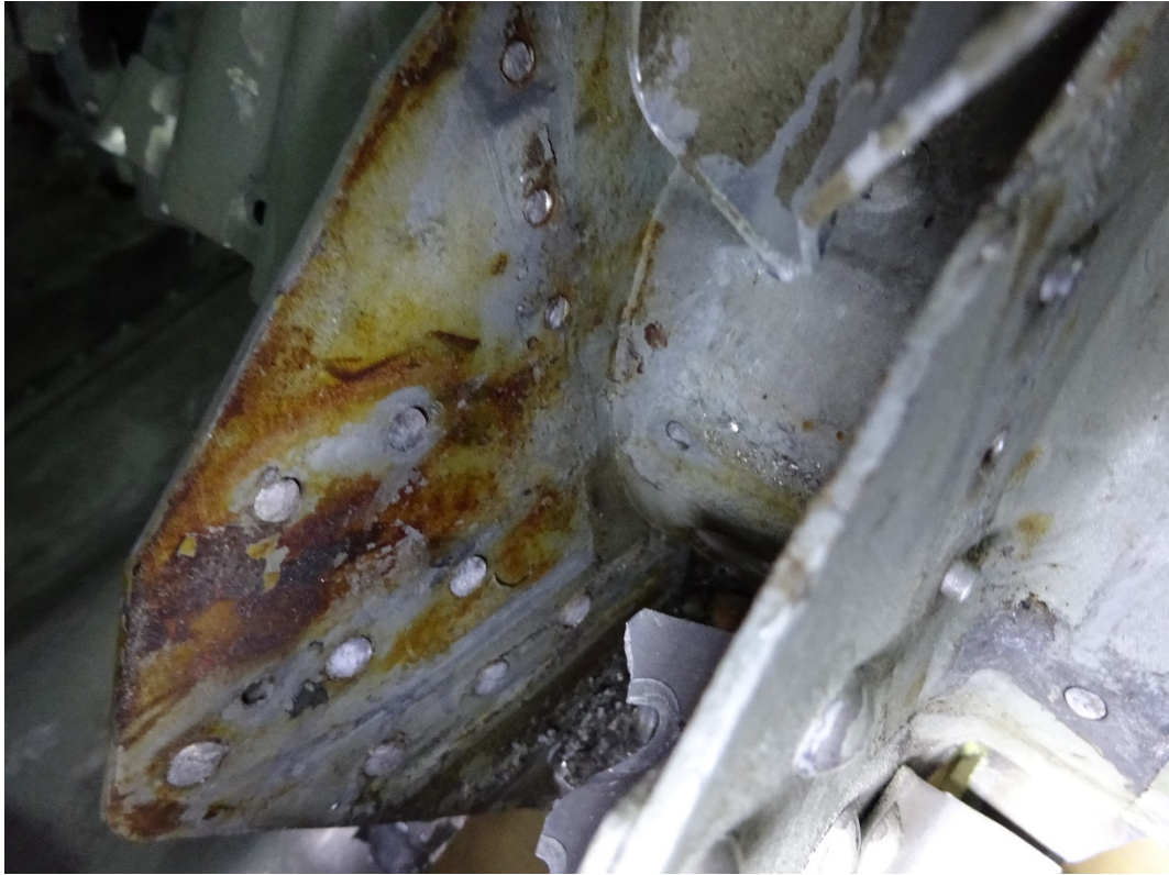
Figure 10: Corrosion in an area connecting the outer wing to the centre wing.
