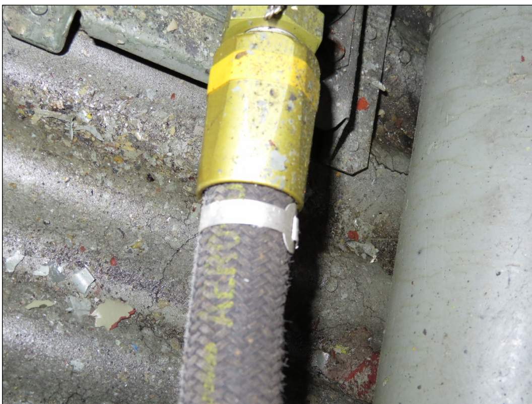
Figure 68: Flaking anti-corrosion paint and severe contamination on the inside of HB-HOP's left-hand outer wing, and fuel line from 1989.
