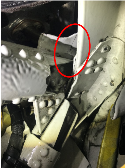
Figure 45: Crack in the mounting frame gusset plate (red circle). Photograph provided by Ju-Air.
