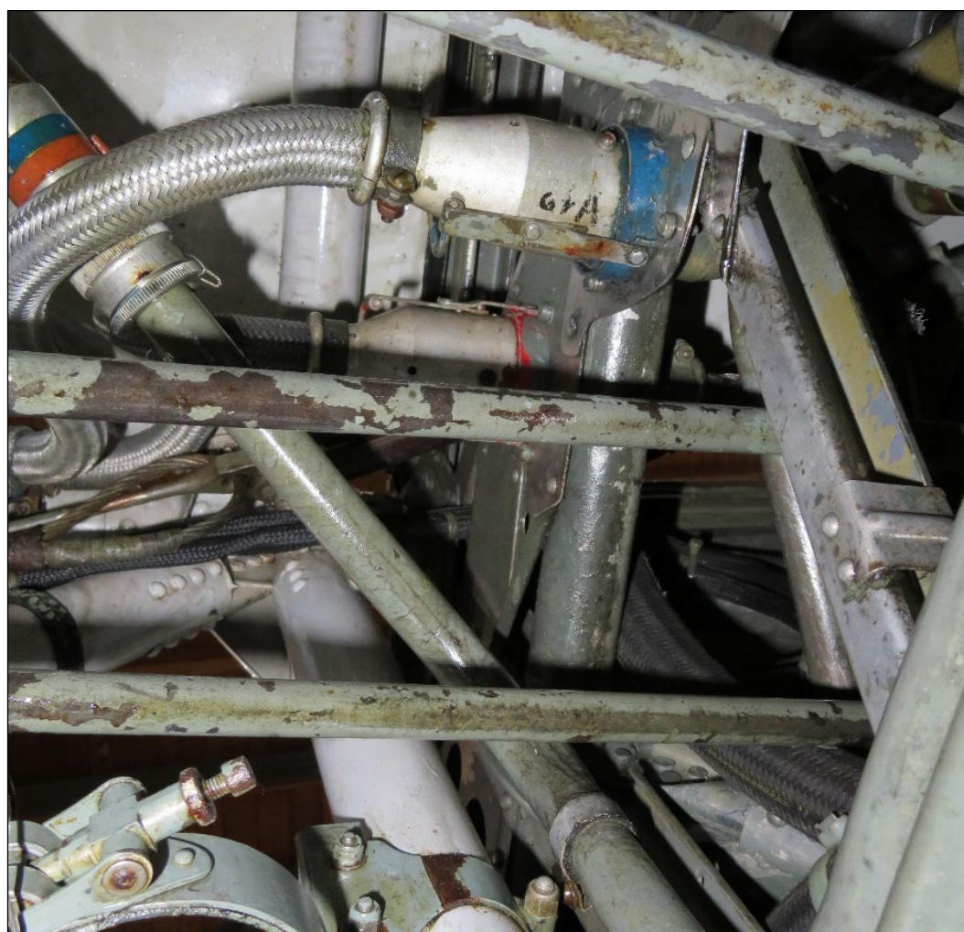
Figure 70: Corroded components and a lack of anti-corrosion paint on the inside of HB-HOP's left-hand outer wing.
