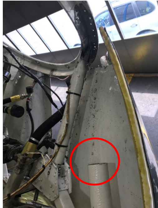
Figure 46: Cut strut tubing (red circle). Photograph provided by Ju-Air.
