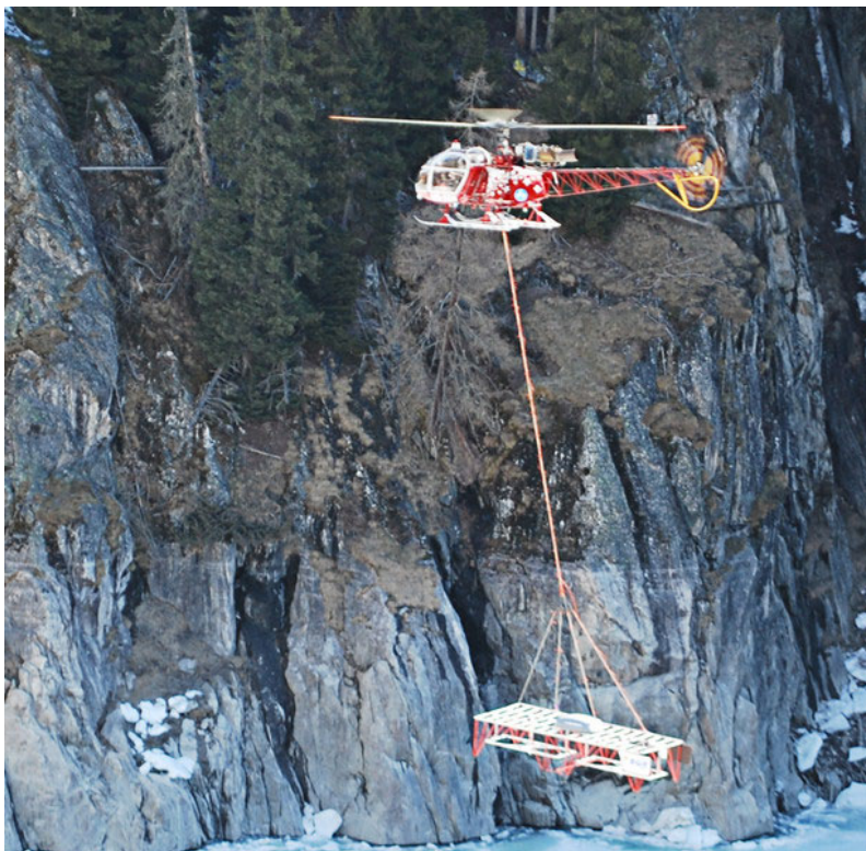
Fig. 36: Hera-G radar system (RST) operated by helicopter
